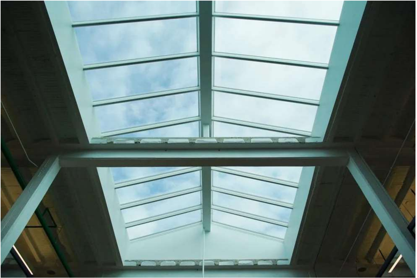
The skylight in the center of the new West Side Bazaar.
