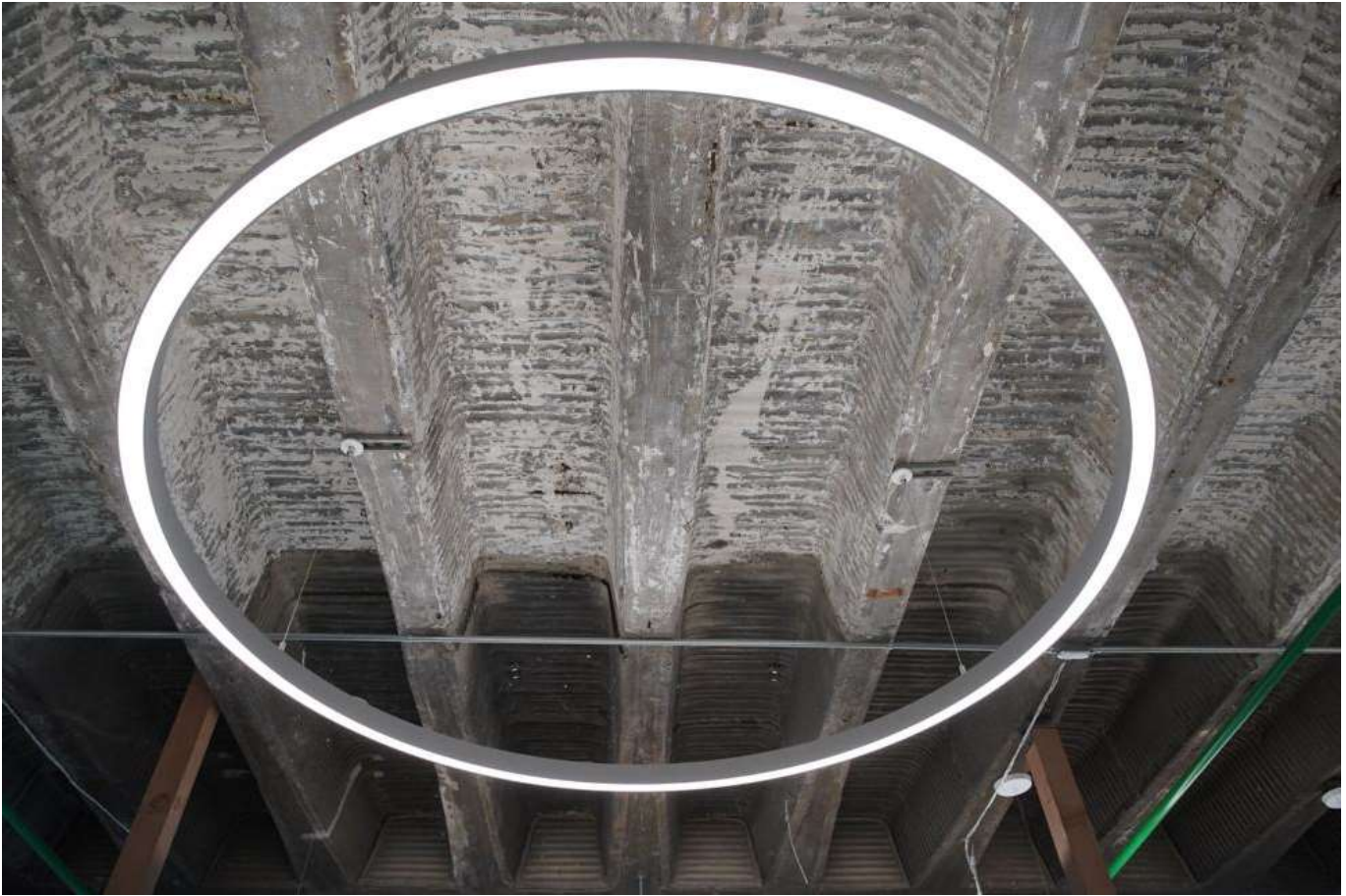
Lighting in a retail booth in the new West Side Bazaar.
